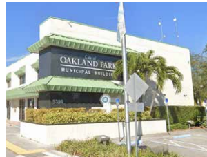
Municipal Building Hardening 5399 North Dixie Highway
