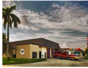
Fire Station 87 Hardening 2100 NW 39th Street
