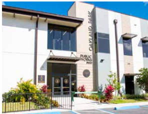
Public Works Facility 5100 NE 12th Terrace
